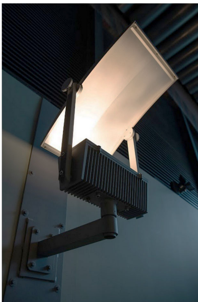
Left: Indirect Post Top Fixtures intended to spill some light onto ceiling and reflect most light back down to task plane
