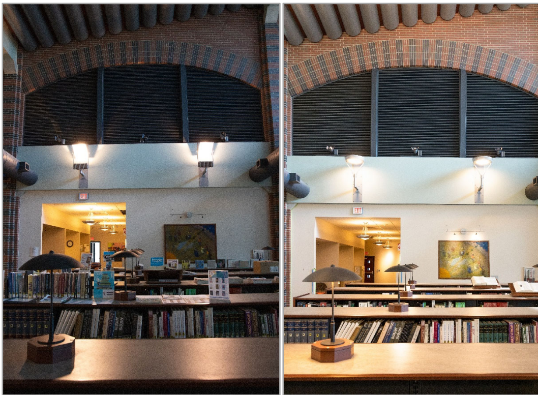
Left / Before: Poor task plane illumination, high glare from operating post tops, no uplight from broken spot luminaires Right / After: 30 foot candles on task plane, balance fixture glare compared to surrounding luminances, balanced uplight
